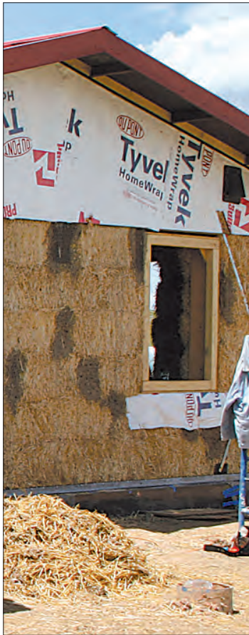
Bales of straw provide good insulation for homes and lay people find them easy to work with.
